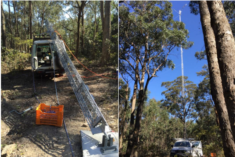
Figure 18. The 30 metre eddy covariance tower erected on a concrete pad in Wombat State Forest, September 2015.
