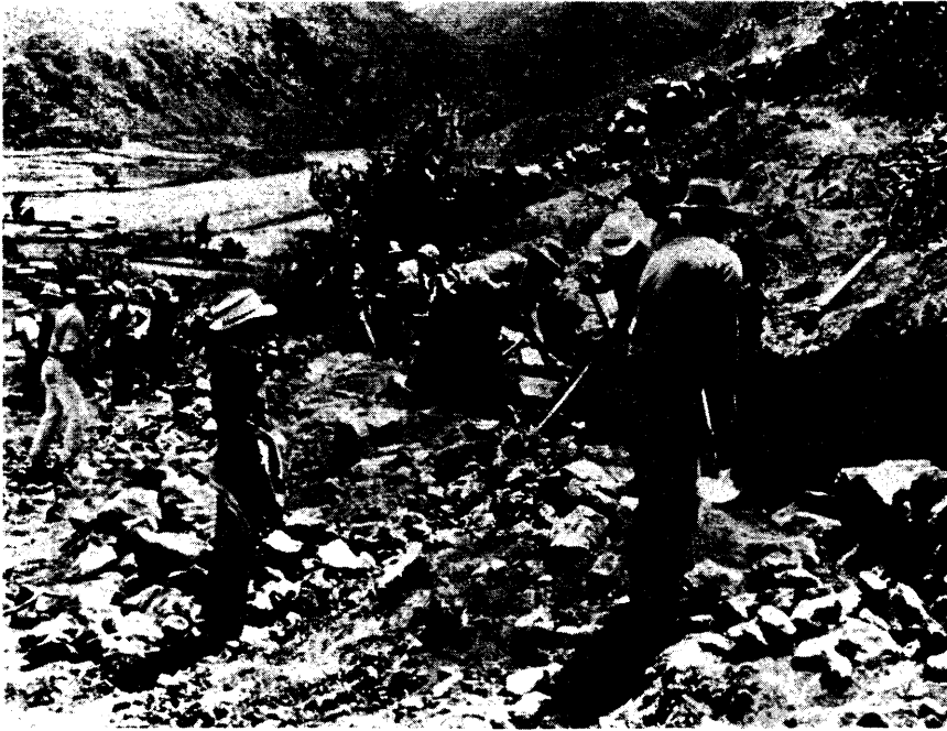
Plate 2 Rebuilding abandoned agricultural terraces in Coporaque, Arequipa, Peru, by placing new wall base stones and building the wall upwards to retain the soil.
